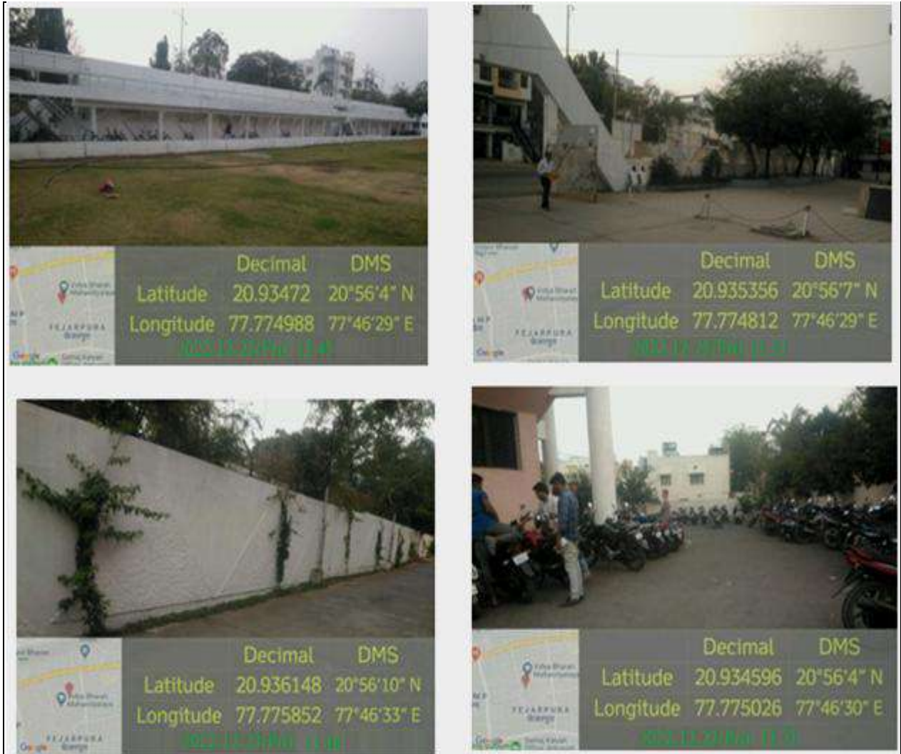
Safety compound walls around the campus
