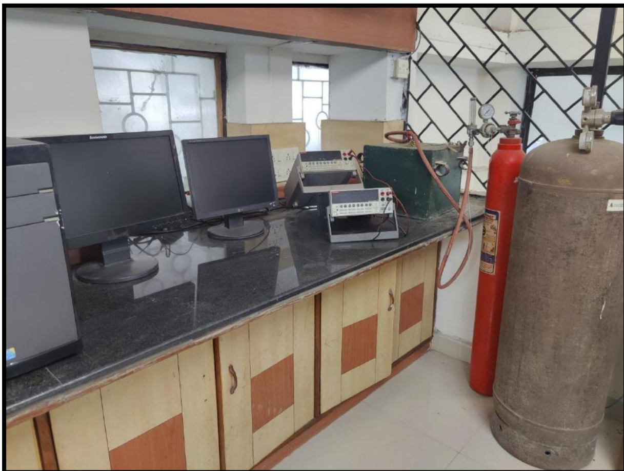
Low gas concentration measuring unit with micro-voltmeter and pico-ammeter interfaced with computer enabled measurement (Department of Physics)
