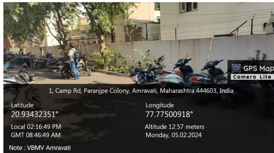
Safety compound walls around the campus
