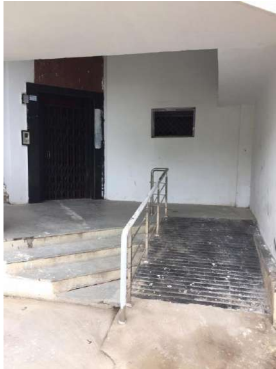
Ramp at Main Building
