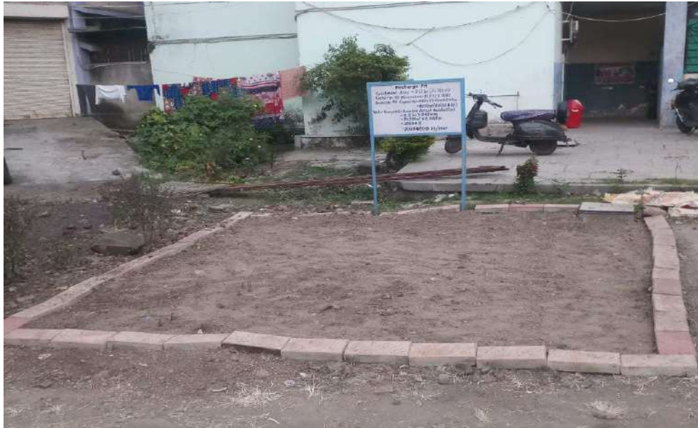
2 Million Liters of Rainwater Harvested every year in a Recharge Pit of 12x12x10ft near borewell
