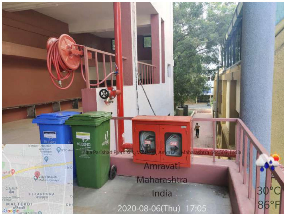
At 2 nd Floor of the Main Building
